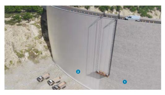
1 Substrate 2 Waterproofing layer KÖSTER TPO Aqua 2.5 Geo
