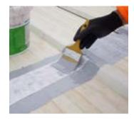
KÖSTER Superfleece can be embedded into the fresh layer on substrates that are at risk of cracking
